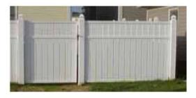
Fences abutting a local residential street must be installed parallel to the street. The fence must be installed no closer than one (1) foot from the sidewalk or eleven (11) feet behind the curb of an intersecting street or edge of an alley.
